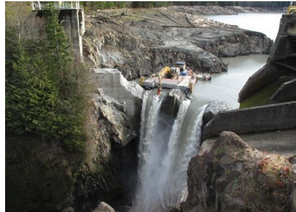
Glines Canyon Dam Removal
